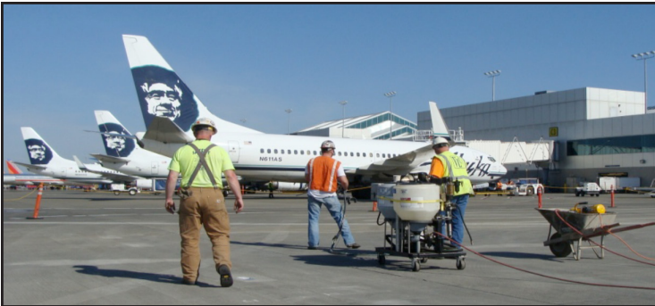
The single operator and a couple of supervisors on the job
